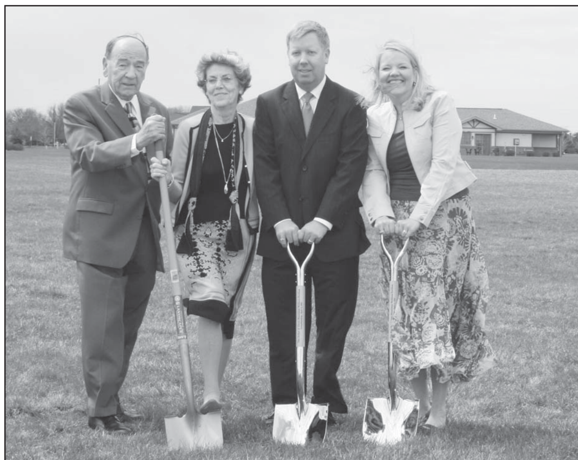
Left to right: Paul Zurcher, Marilyn Muselman, Roger Muselman and Karen (Muselman) Thomas take part in the groundbreaking ceremony marking the start of construction of the Arthur and Gloria Muselman Wellness Pavilion at Swiss Village on Friday. [Photo by Linda Quinlan]
